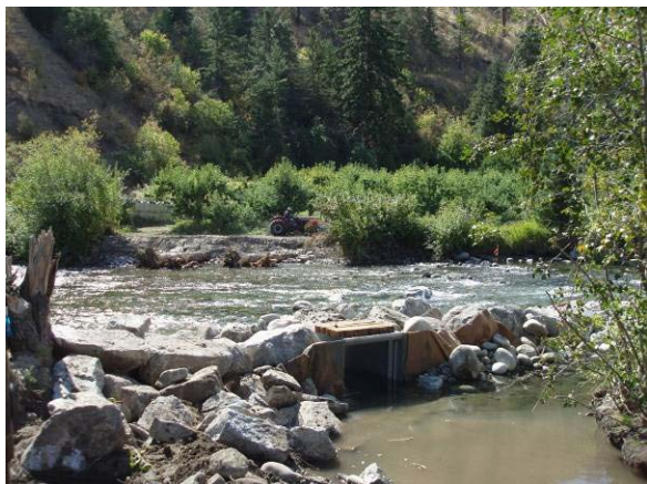
Photo 3. Low-height diversion rock barb on river left across from root wads shown in previous photos.
