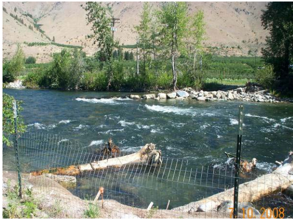
Photo 1. Two root wads keyed into the bank river right in the foreground and across the river on the left bank is a low-height diversion rock barb with sluice gate for a point of diversion at river mile 2.9. The river is moving to the east left to right.
