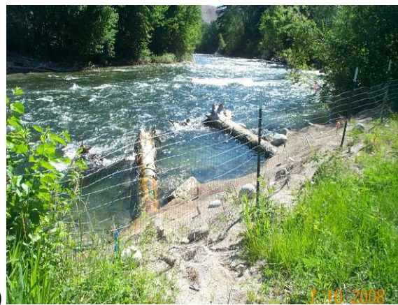
Photo 1. Two root wads keyed into the bank river right in the foreground and across the river on the left bank is a low-height diversion rock barb with sluice gate for a point of diversion at river mile 2.9. The river is moving to the east left to right.
