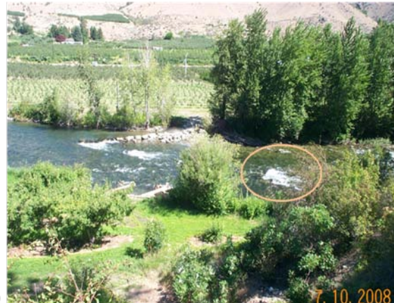
Photo 3. Low-height diversion rock barb on river left across from root wads shown in previous photos.
