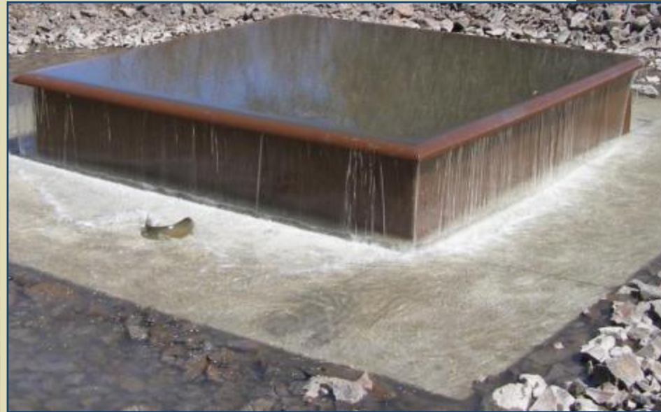
NRCS design to prevent fish entrapment
